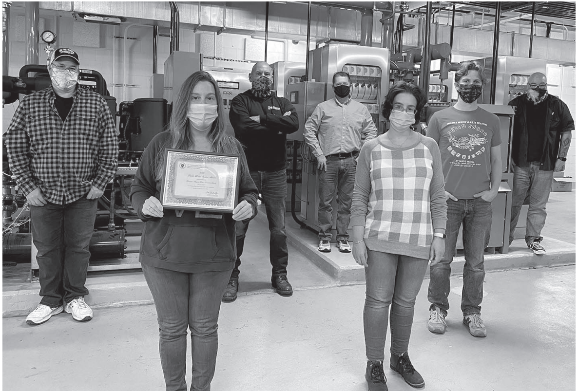
Filtration plant staff in front of the new ozone generators holding the Mass EPA award.
